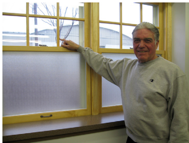
Russ explains the construction of the true divided light windows A-Craft recently manufactured and installed in their own building.
